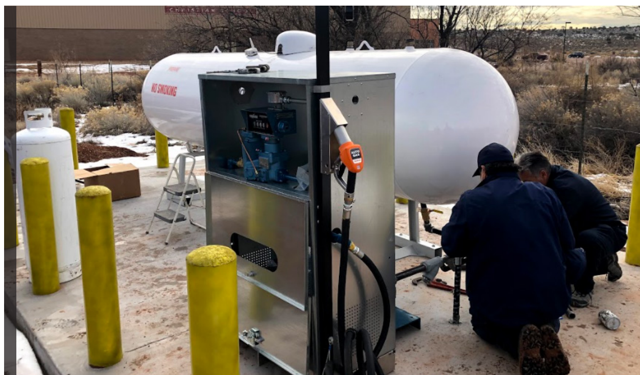
Left: The new propane fueling station being installed on campus.
